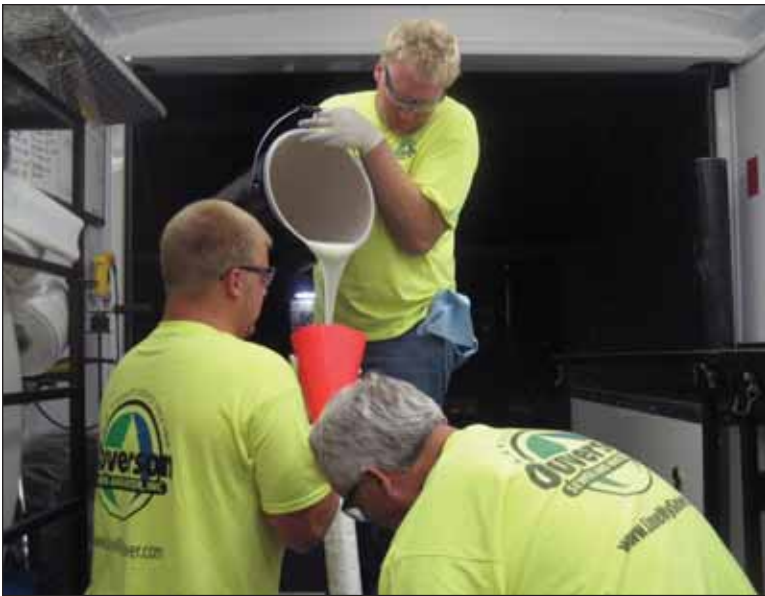
Troy Ouverson pours resin into a cone to begin the wetting-out process. Scott Veal holds the cone and Doug Ouverson assists him.
